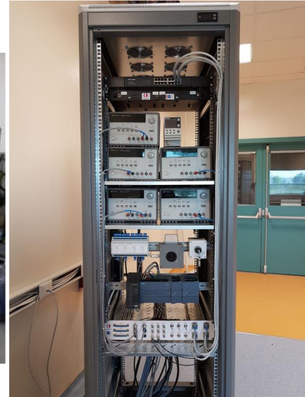
Power supplies and cabling → For powering up, communicating with electronics of the beamline
