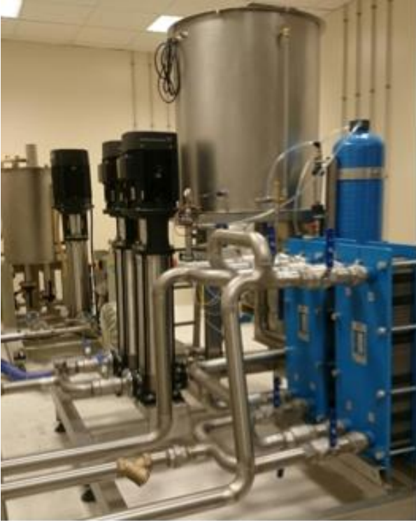
Cooling system → To cool down magnets and collimators
